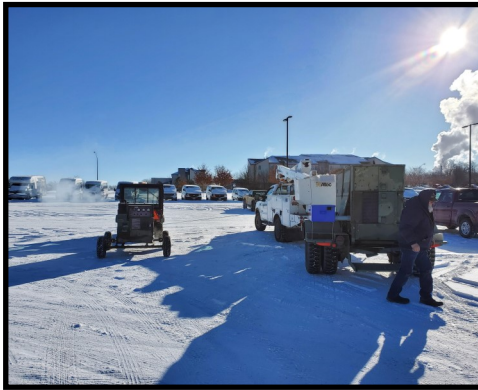
Preparing generators for possible shutdown
